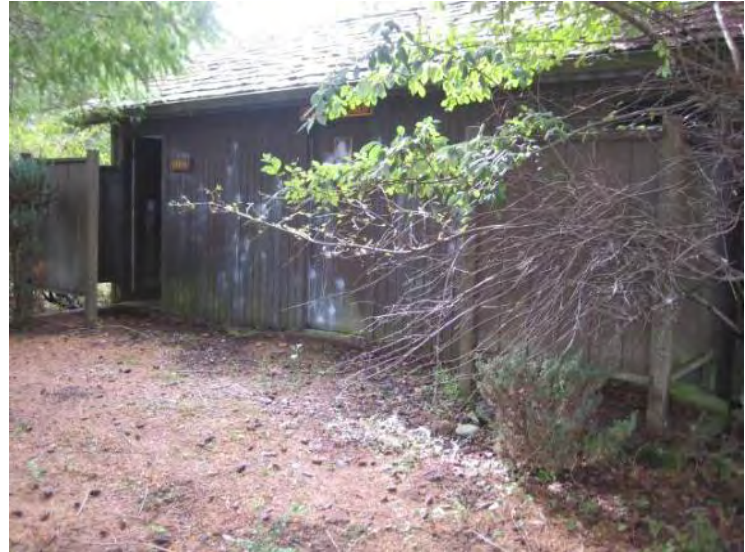
Photograph 8 Sanitary stations located throughout Section 1
