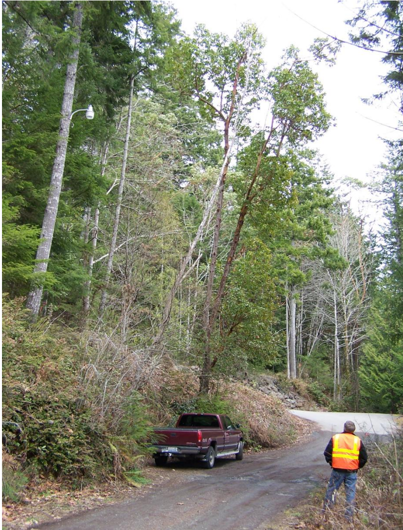
Figure 06 Image #2708 / Dead tree overhanging parking area near the east end of MC-4 Photo: RMG
