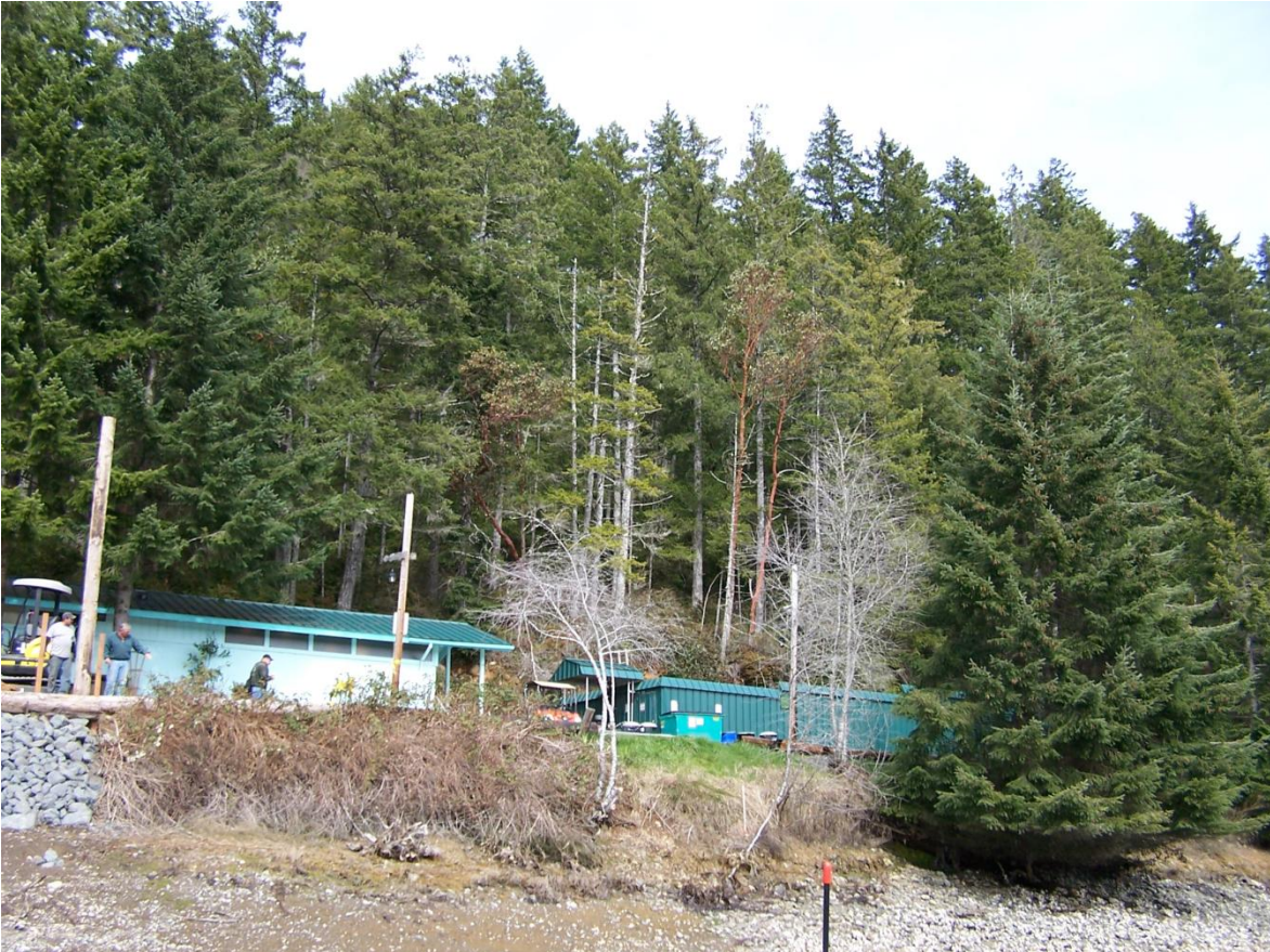
Figure 05 – Image #2662/ Dead trees behind and overhanging buildings / Photo: RMG
