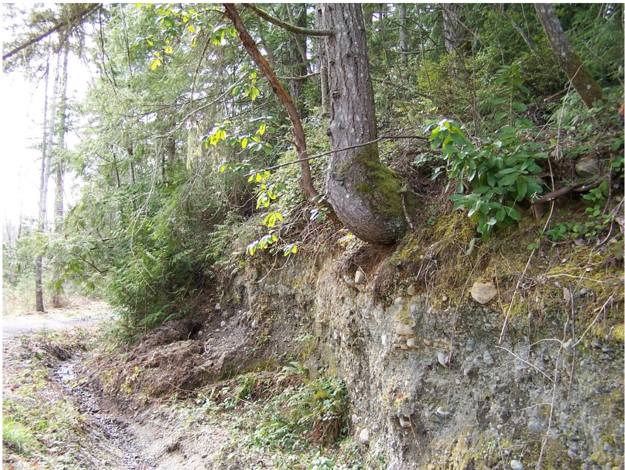
Figure 11 / Image #2800 / Tree at cut bank edge overhanging single family home parking area / Photo: RMG
