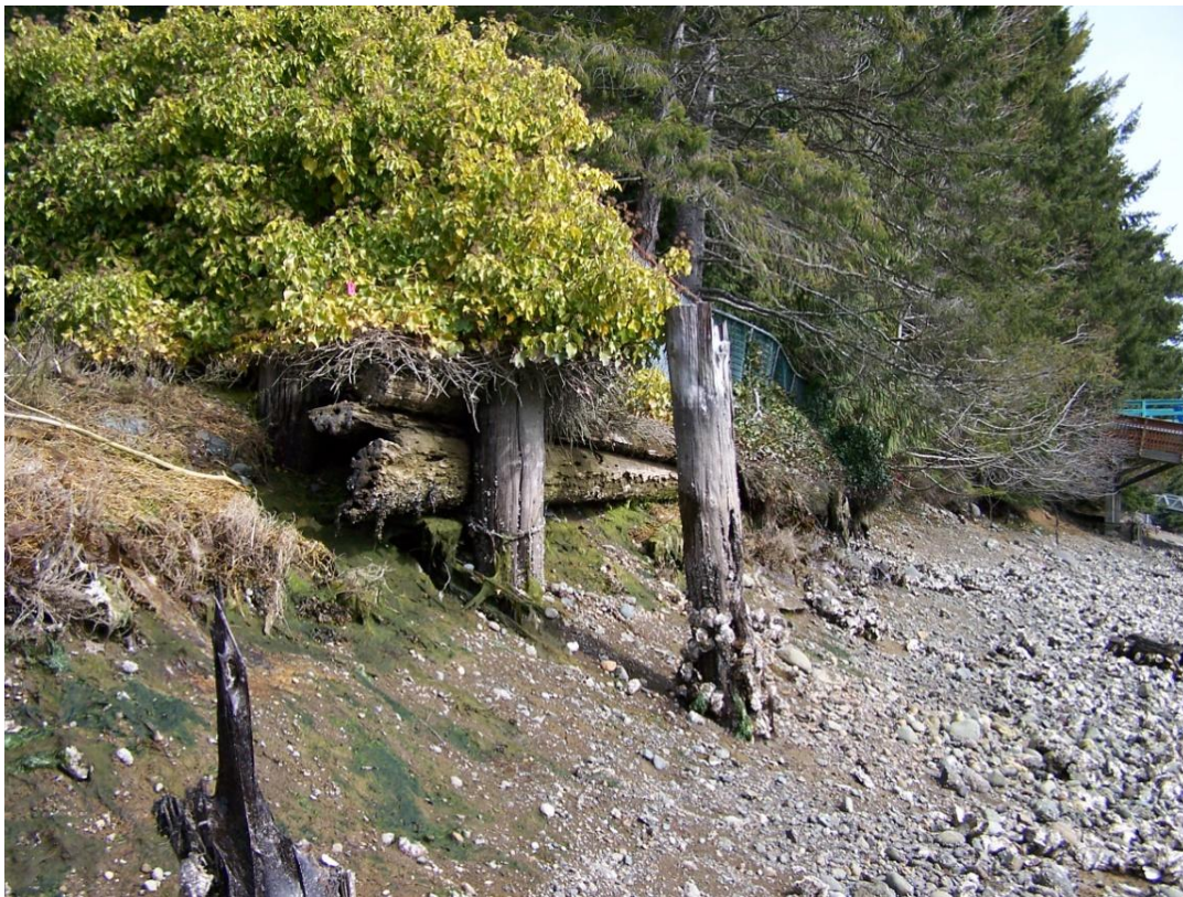
Figure 14 / Image 2648 / Remaining pilings and bulkhead from historical log dump operation / Photo: RMG
